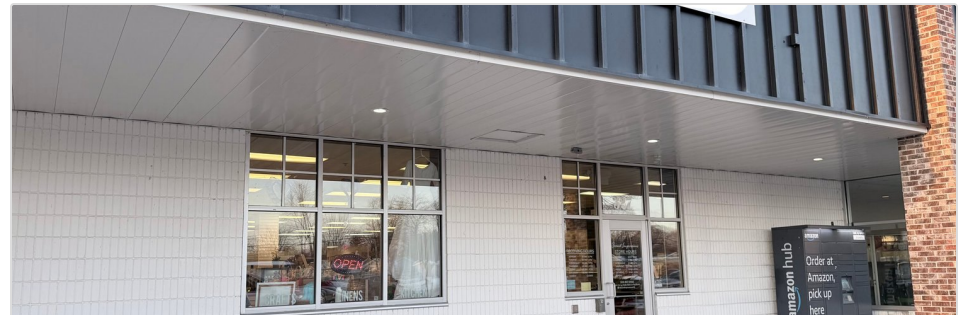
STOREFRONT ENTRANCE & AMAZON HUB PICKUP
